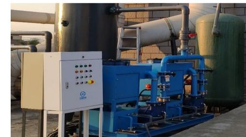
Tunnel oven uses heat pump for energy saving. The oven electric heater was replaced with a condenser, using a heat pump for heating and heat exchange, achieving an annual power saving of 310,000 kWh, and a carbon reduction of 178 tonnes of CO<sub>2</sub> equivalent.
