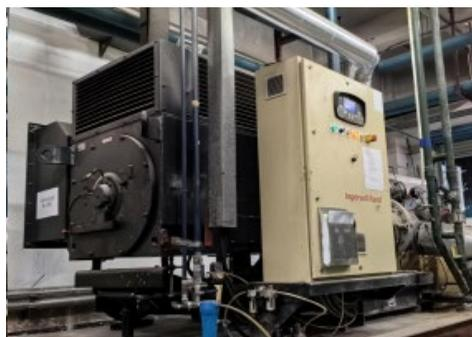
Air conditioning system energy saving. Using waste heat hot water and high-pressure micro-mist to replace traditional electric heater hot water steam humidification, after the transformation, the efficiency increased by 90%, the annual power saving was over 1.52 million kWh, and the carbon reduction was 886 tonnes of CO<sub>2</sub> equivalent.
