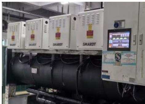
Air pressure system energy saving. The old screw air compressor was replaced with a 10KV high-pressure centrifugal air compressor, efficiency was increased by more than 20%, the system's annual power saving was 2.28 million kWh, and annual carbon reduction was 1,324 tonnes of CO<sub>2</sub> equivalent.
